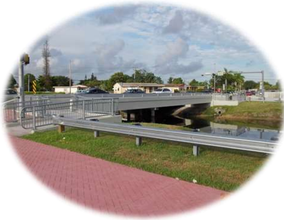
School Safety Bridge
